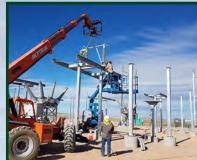
be constructed after NTUA assumes ownership. As a result – a new switching station was constructed and was put into service in December 2017. This allows NTUA to switch electric load in the event of a regional outage, keeping electric services to areas not directly affected by the outage.
